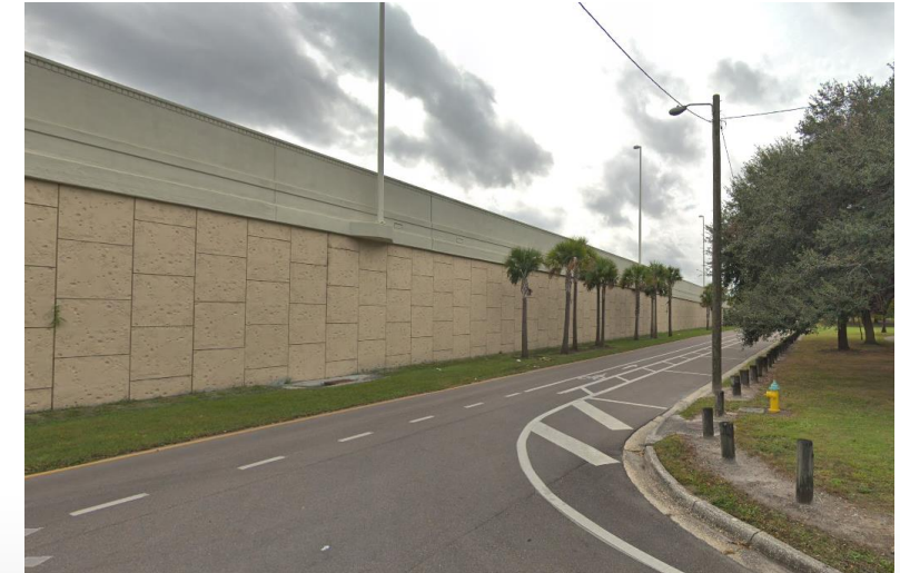
Recent improvement: mainline elevated without fencing along LA R/W
