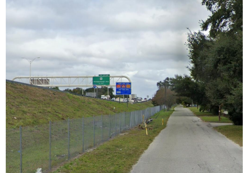
Existing project: mainline elevated with fencing along LA R/W
