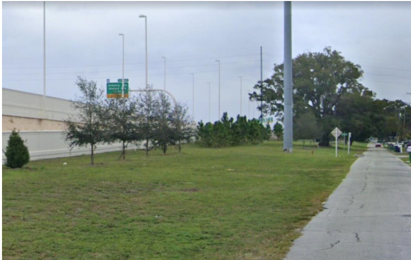
Recent improvement: mainline at-grade without fencing along LA R/W
