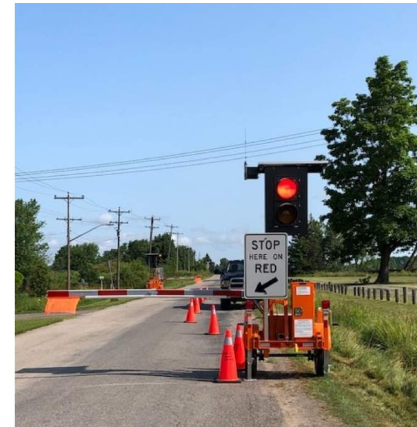
AUTOMATED FLAGGER ASSISTANCE DEVICES (AFAD) ARE TEMPORARY TRAFFIC CONTROL EQUIPMENT.
